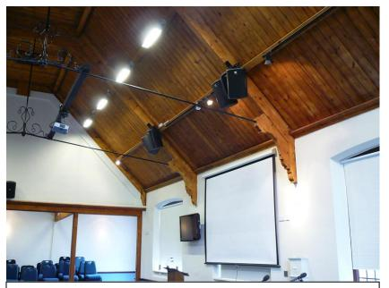
Ceiling mounted EV ZX1i speakers for landscape orientation. The main projection screen and wall mounted LCD displays are also visible.
